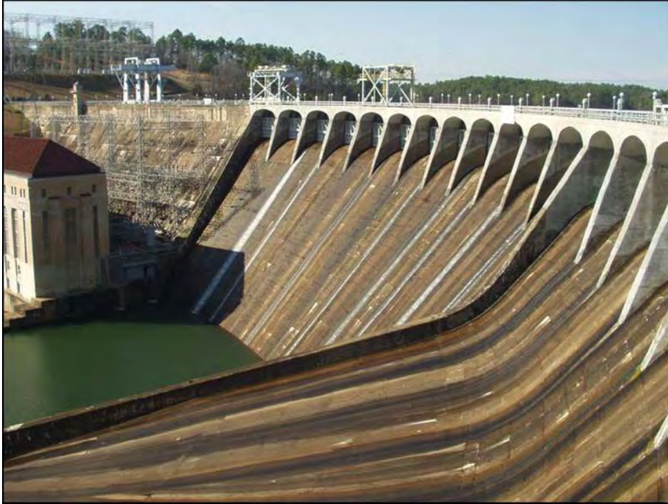
PHOTO 4-3 DOWNSTREAM VIEW OF MARTIN DAM
