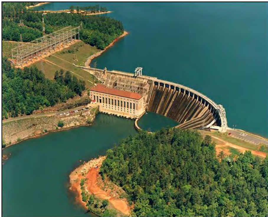
PHOTO 4-2 AERIAL VIEW OF MARTIN DAM AND POWERHOUSE
