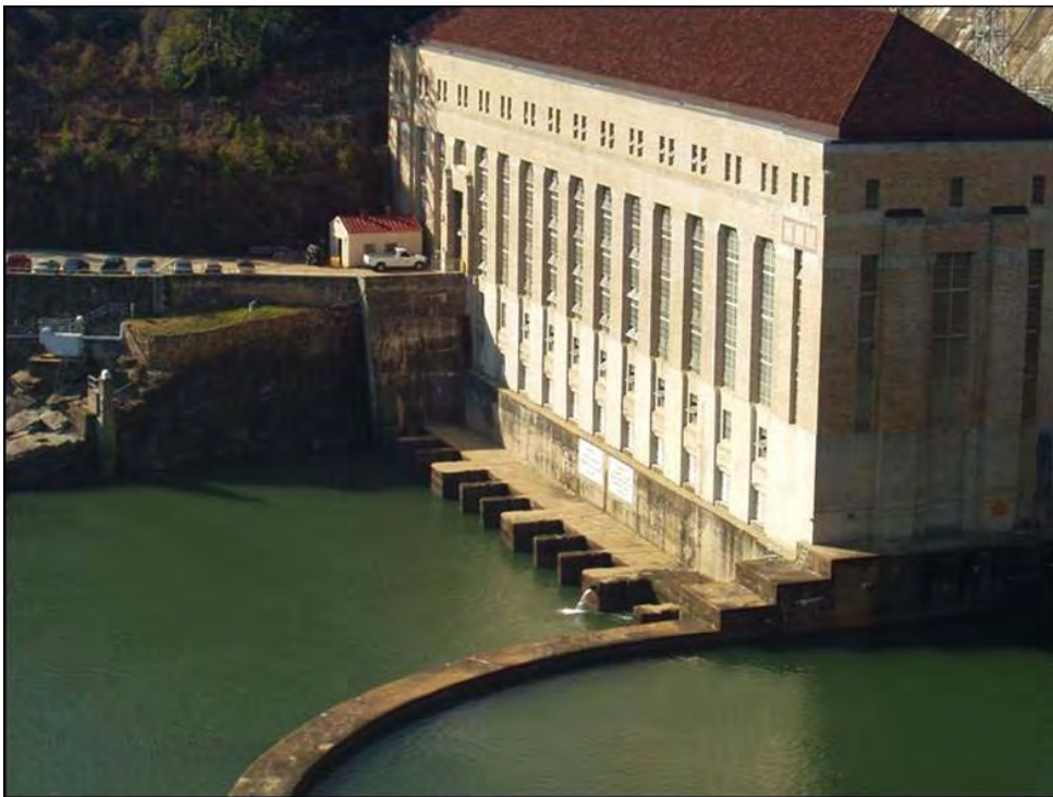
PHOTO 4-4 MARTIN POWERHOUSE, AS VIEWED FROM EAST SIDE OF DAM
