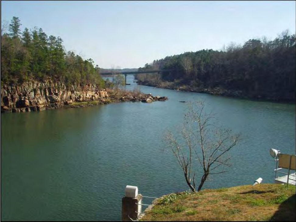
PHOTO 4-5 DOWNSTREAM VIEW OF TAILRACE
